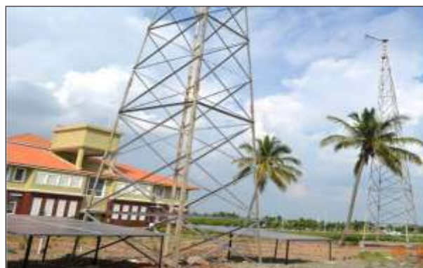
7. Wind & Solar Hybrid System for Generating Electricity
