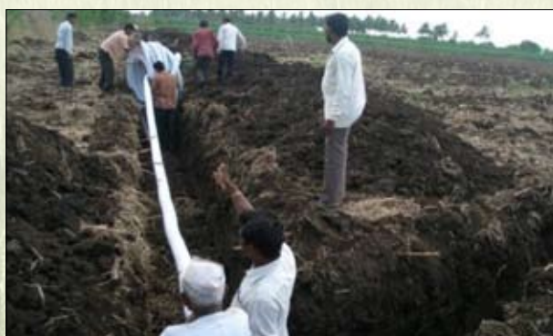
Reclamation of Problematic Soils By Using Subsurface Drainage and Mole Plough
