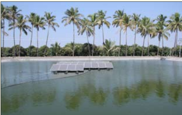
Water Storage Tanks with solar water lifting system
